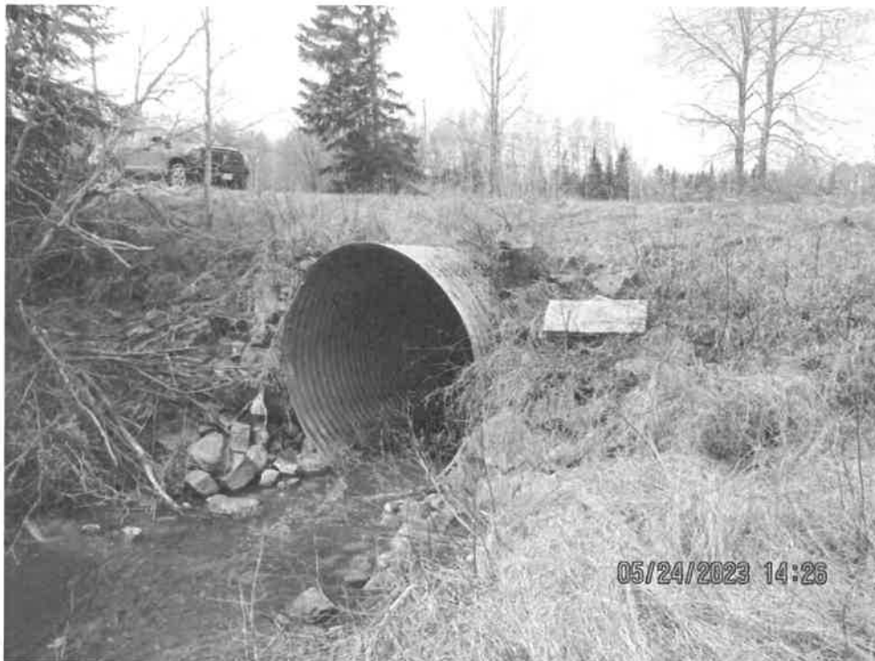
Photo 4: South end (outlet) of culvert.
