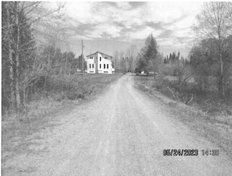
Photo 1: East approach to culvert.
