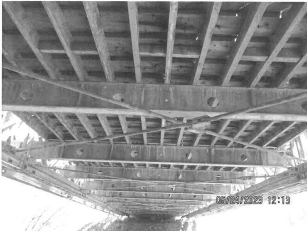
Photo 14: Underside of deck (typ.).
