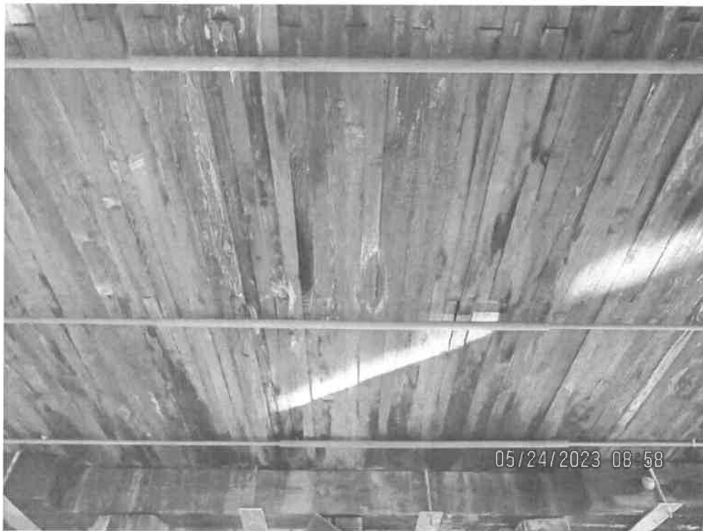
Photo 14: Deck underside (typ.).
