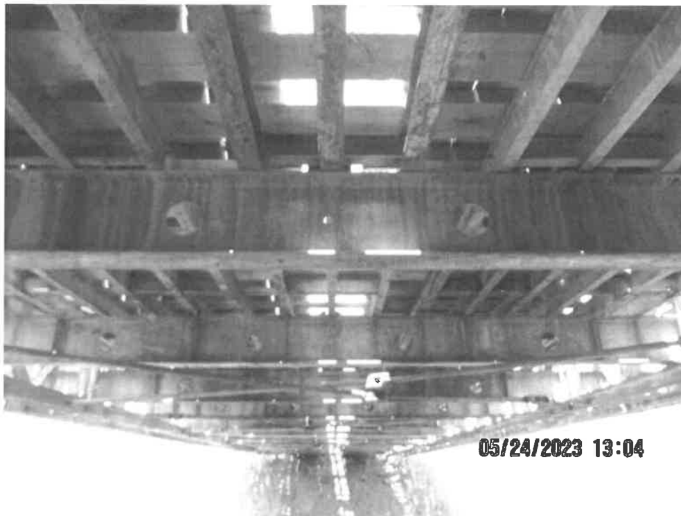
Photo 14: Underside of deck (typ.).
