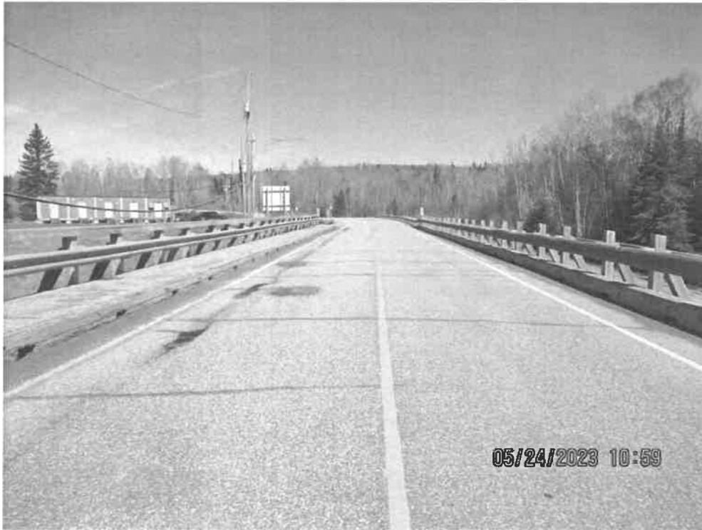
Photo 11: Deck cross section.
