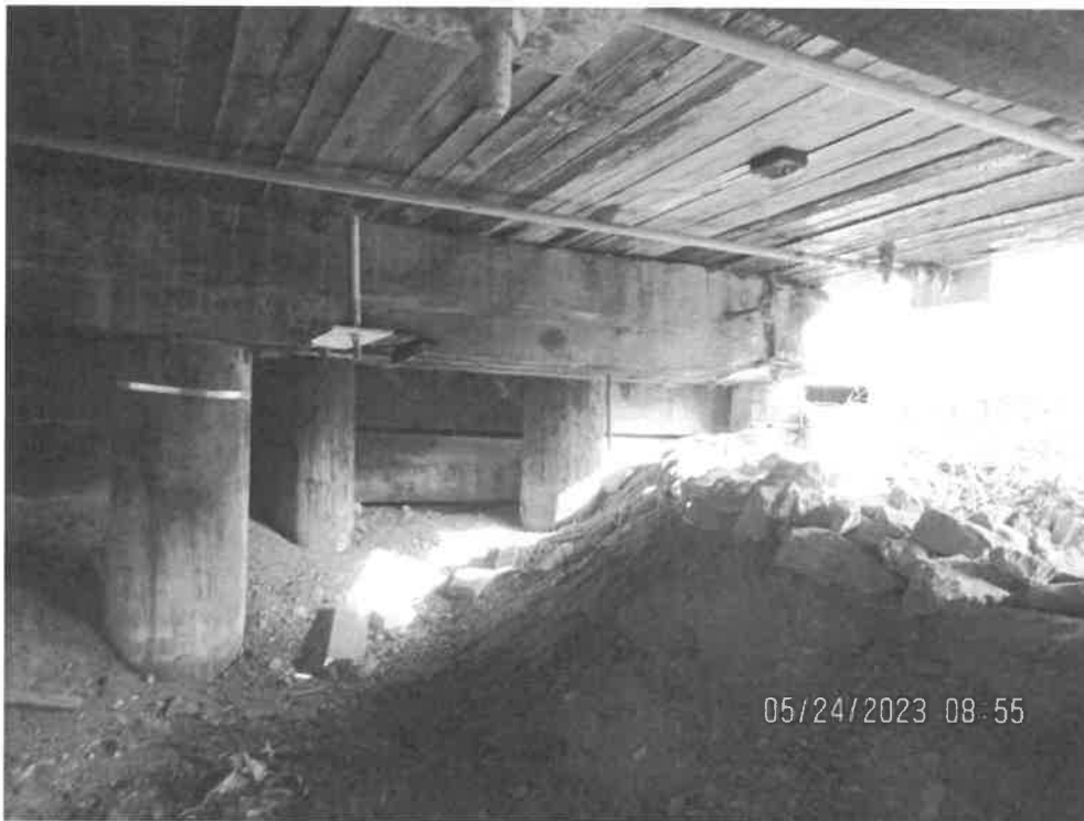
Photo 26: First pile from east removed at Bent #14.
