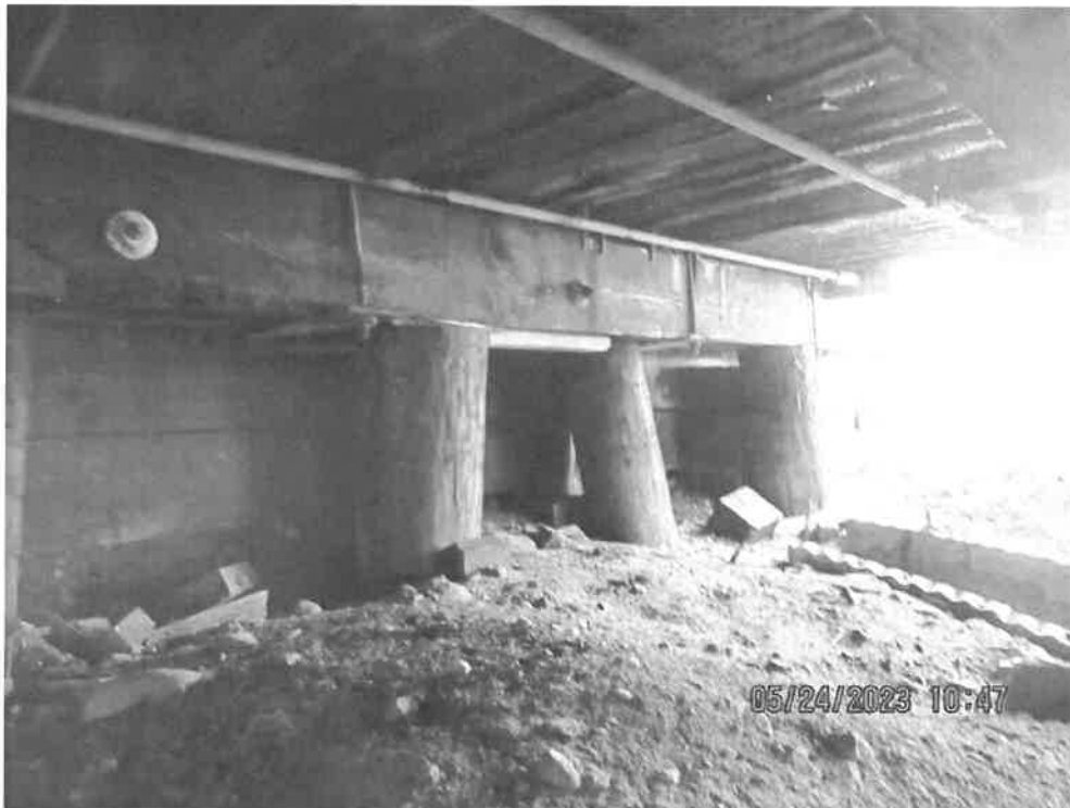
Photo 28: Approximately 50% contact at two piles at the south abutment (9 th and 10 th pile from east).
