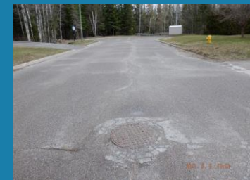
Areas of Construction and Relining
