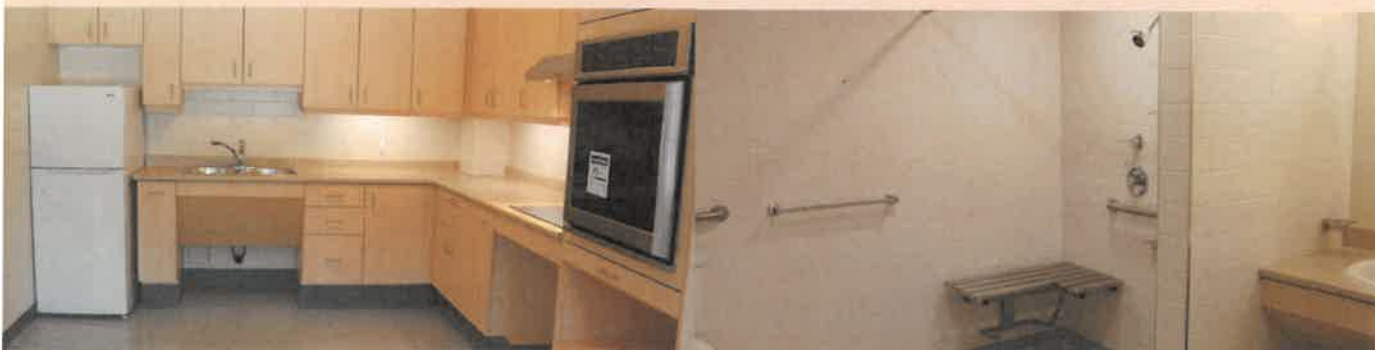
Each unit includes a custom-designed accessible kitchen (LEFT) and a fully tiled bathroom with roll-in shower (RIGHT)
