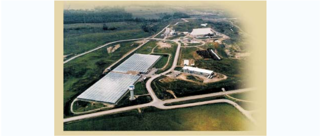
Figure 30– Aerial View of Bruce Eco-Industrial Park
